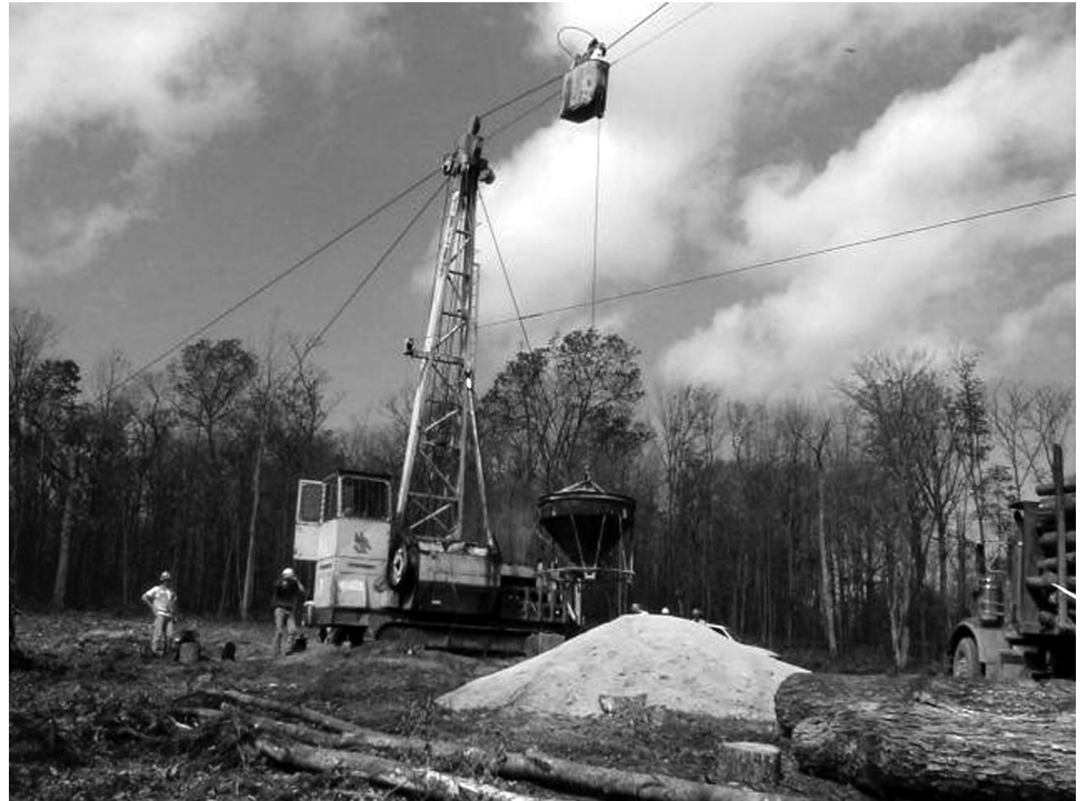
Figure 4: Limestone to Be Added to a Creek to Reduce Acidity at the Burns Creek Pilot Project, George Washington-Jefferson National Forest
